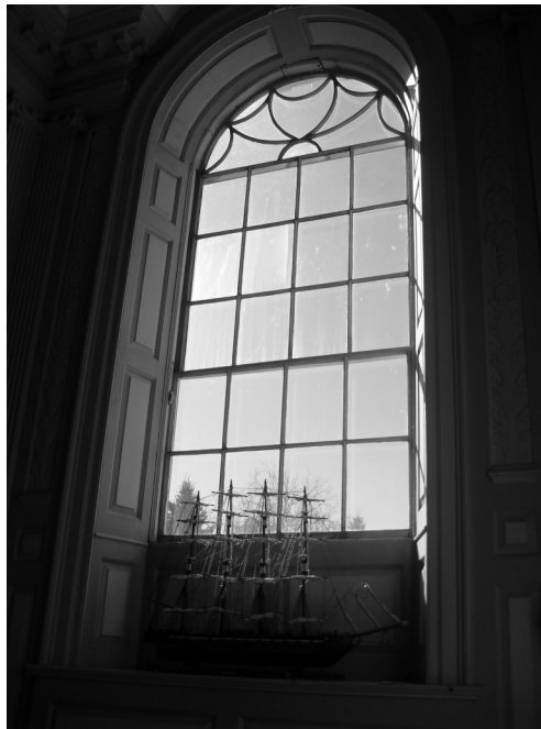
Palladian window in WG House. Photo by Stacey Fraser-deHaan.
